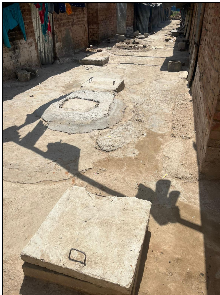
Photograph showing Septic Tank
