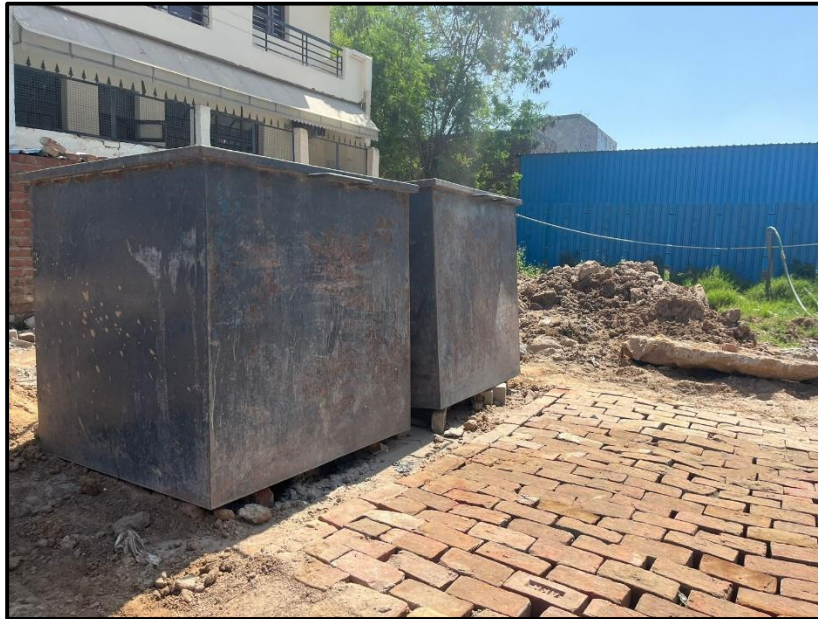
Photograph showing Septic Tank
